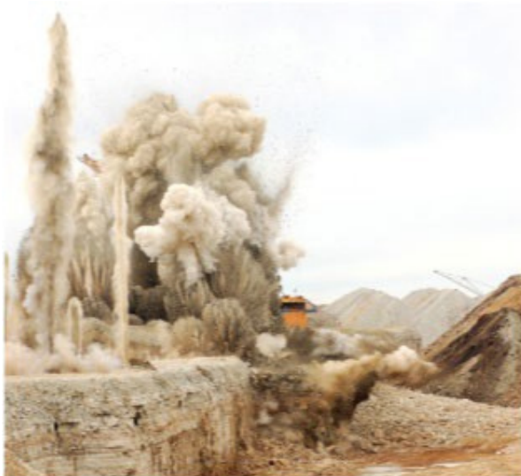
Blasting near the ROW
