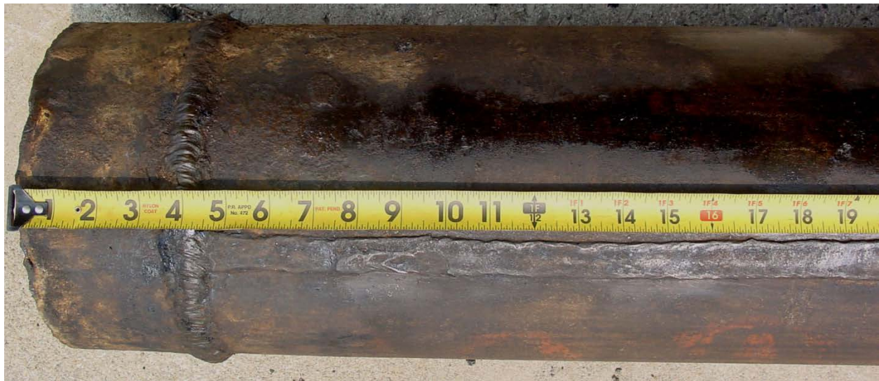
Figure 4. Typical External Appearance of SMAW Seam
