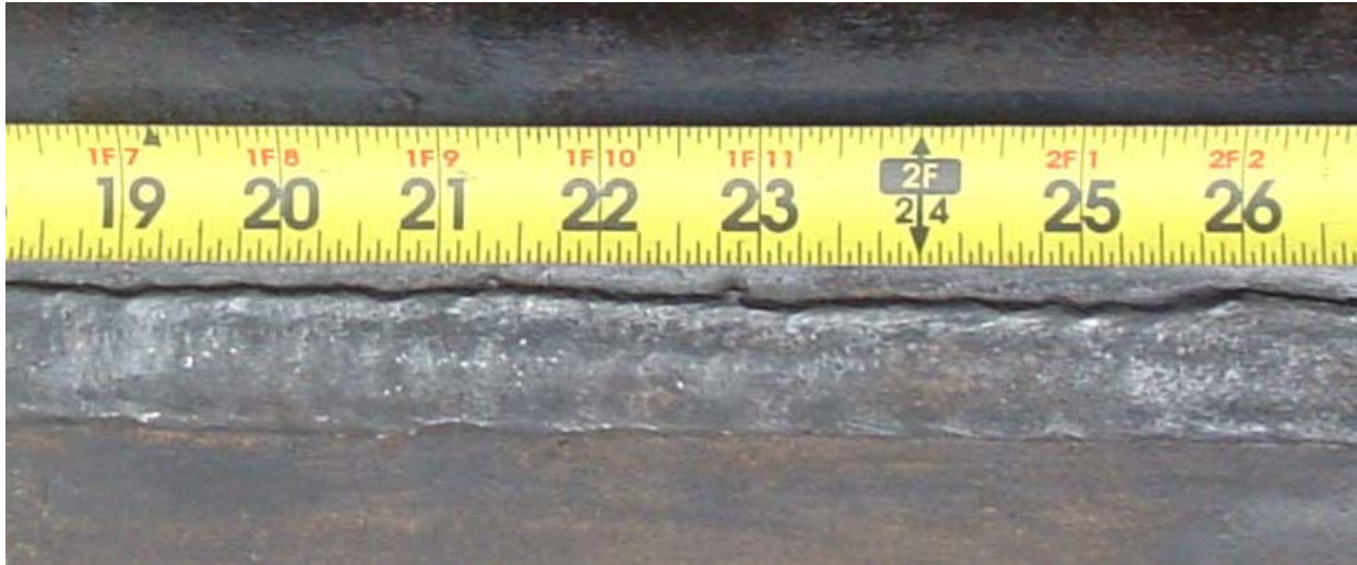
Figure 5. Typical External Appearance of SMAW Seam
