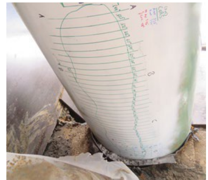
Mechanical dead leg with 6-O'clock position trough type corrosion. From AMPP C 2023-19041 Paper.
