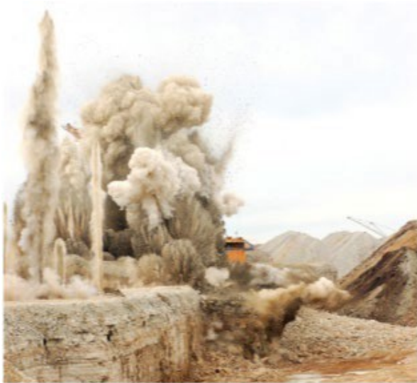
Blasting near the ROW
