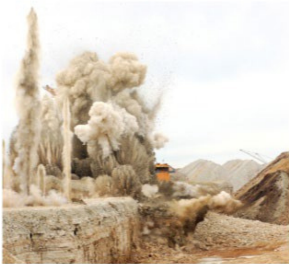
Blasting near the ROW
