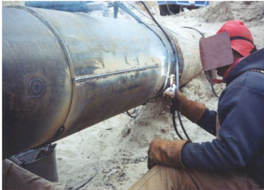
Figure 16. Installation of a Type B repair sleeve.
