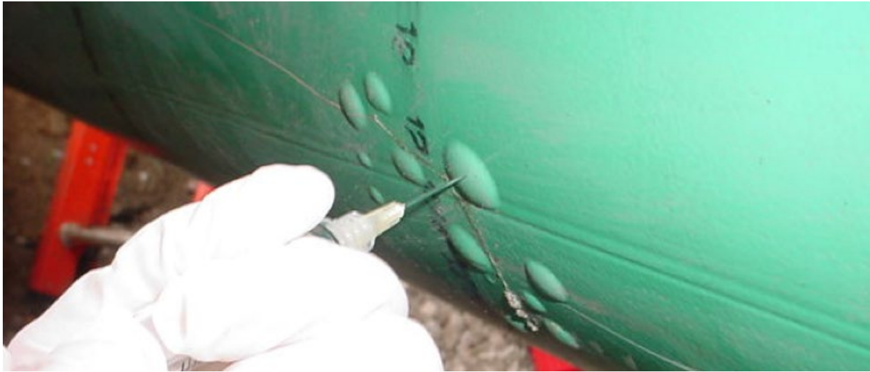
Figure 21. Example of FBE Coating Blisters [40]
