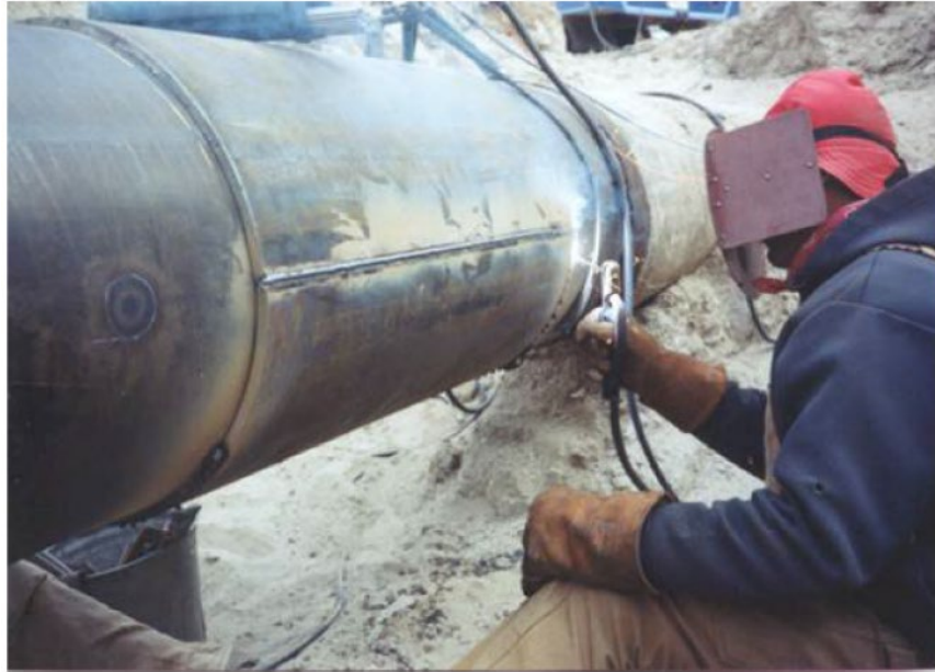
Figure 16. Installation of a Type B repair sleeve.
