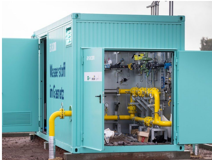
Figure 44. Equipment for Blending H 2 Into NG 83
