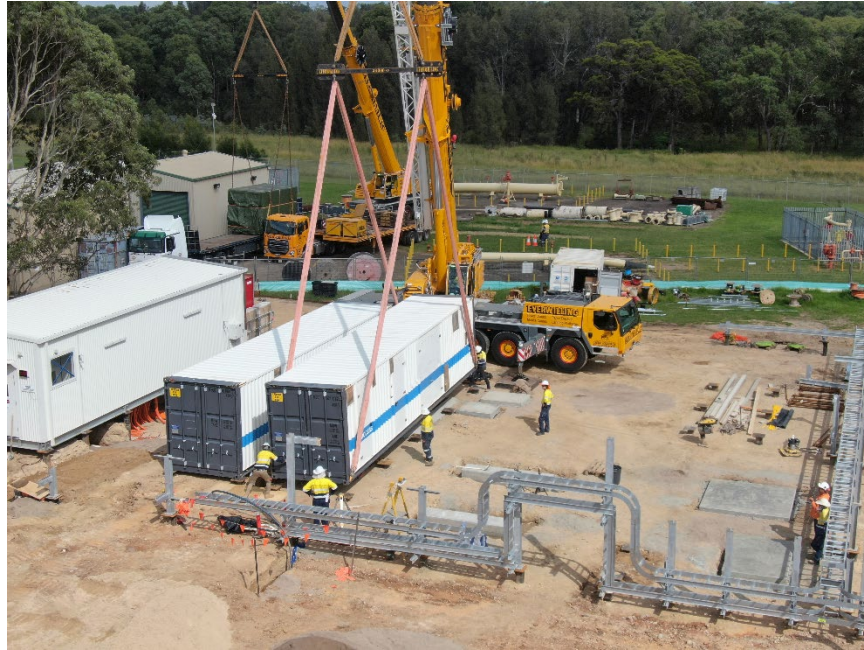
Figure 32. Delivery of Electrolyzers for Western Sydney Green Gas Project, Australia 57
