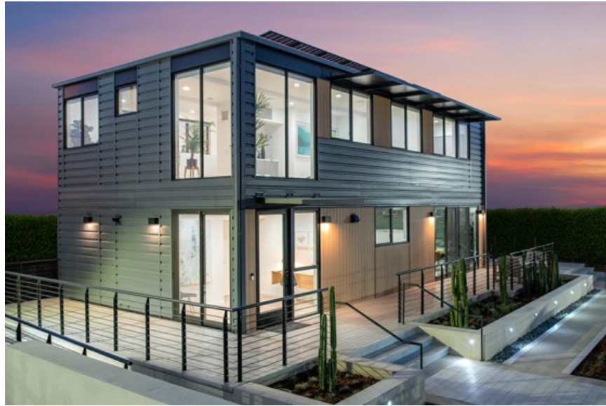
Figure 48. [H 2 ]IE Home in Downey, California 91
