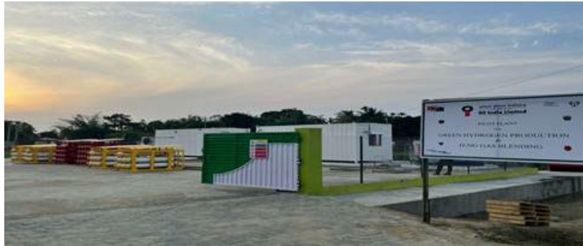
Figure 79. H 2 Facility at Jorhat Pump Station, Assam, India 152
