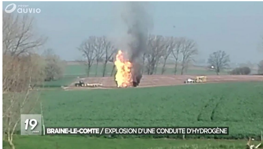
Figure 52. Screen Capture of Video Showing Fire After H 2 Pipeline was Hit by an Excavator
