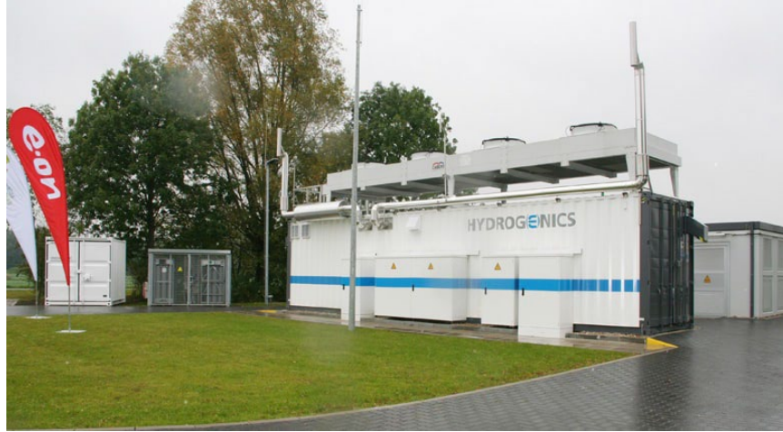
Figure 37. Electrolyzer of PtG Project in Hamburg-Reitbrook, Germany 65
