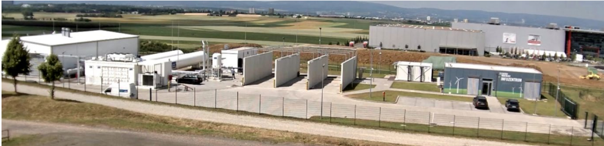
Figure 38. Energiepark in Mainz-Hechtsheim, Germany 67
