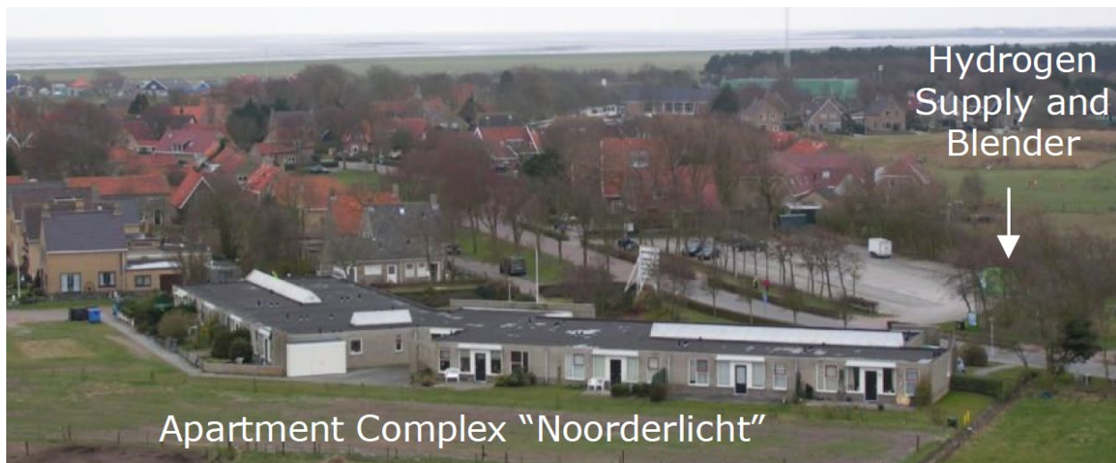
Figure 41. The Hydrogen Supply, Blender, and Apartment Complex "Noorderlicht" on Ameland Island 74
